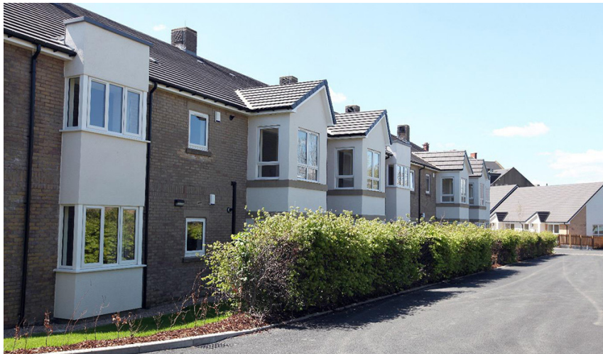
Image of the remodelled elevations with new projecting bay enclosures providing comfortable living spaces to the apartments and increased articulation and visual interest to the elevations.
