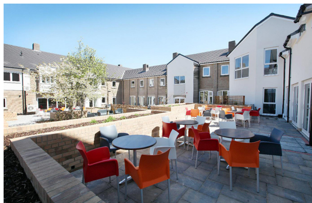
Image of the remodelled external courtyard linked to the internal communal spaces.
