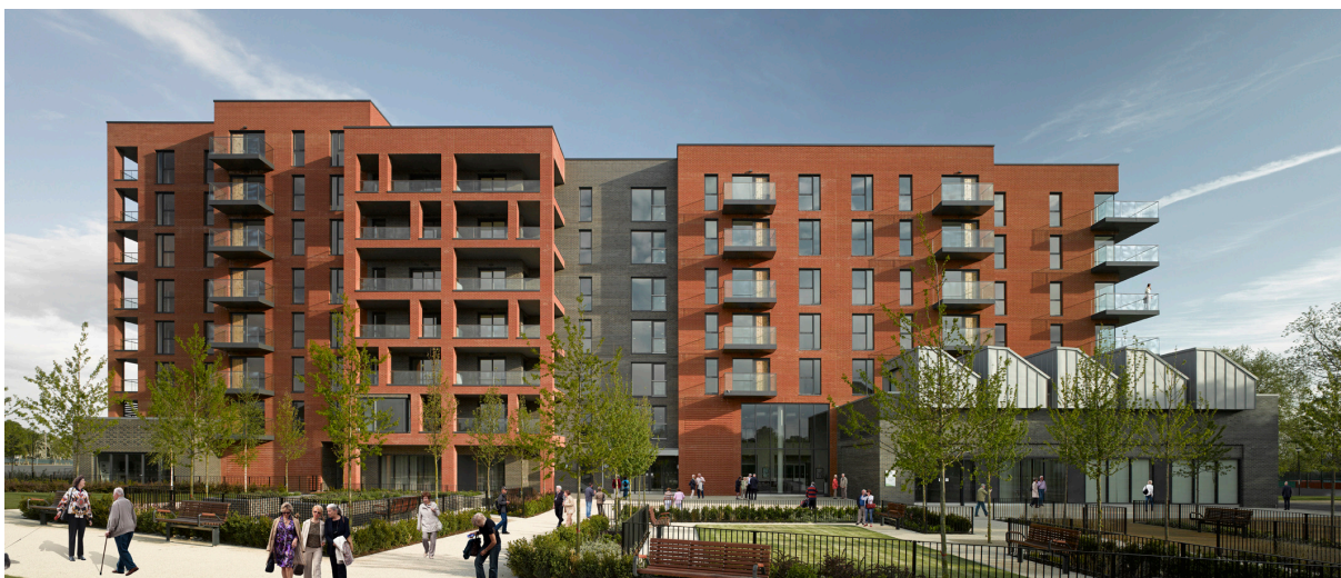
Kidbrooke Village hall, to the right of the main entrance to Halton Court
