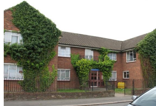
Gresham House, New Malden
