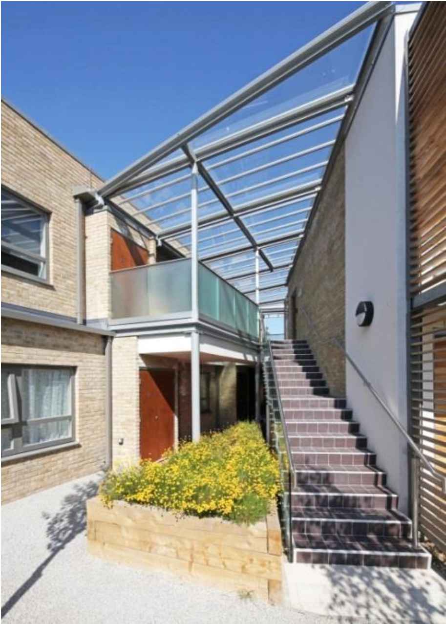
Gresham House, New Malden
