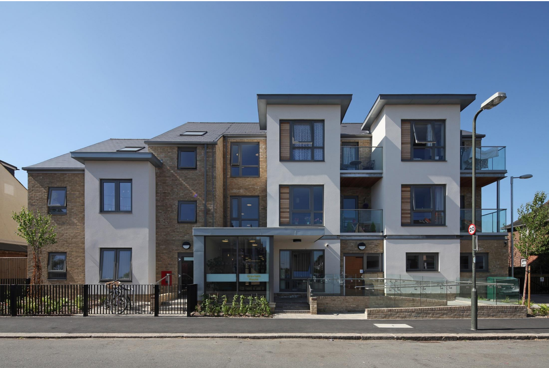
Gresham House, New Malden
