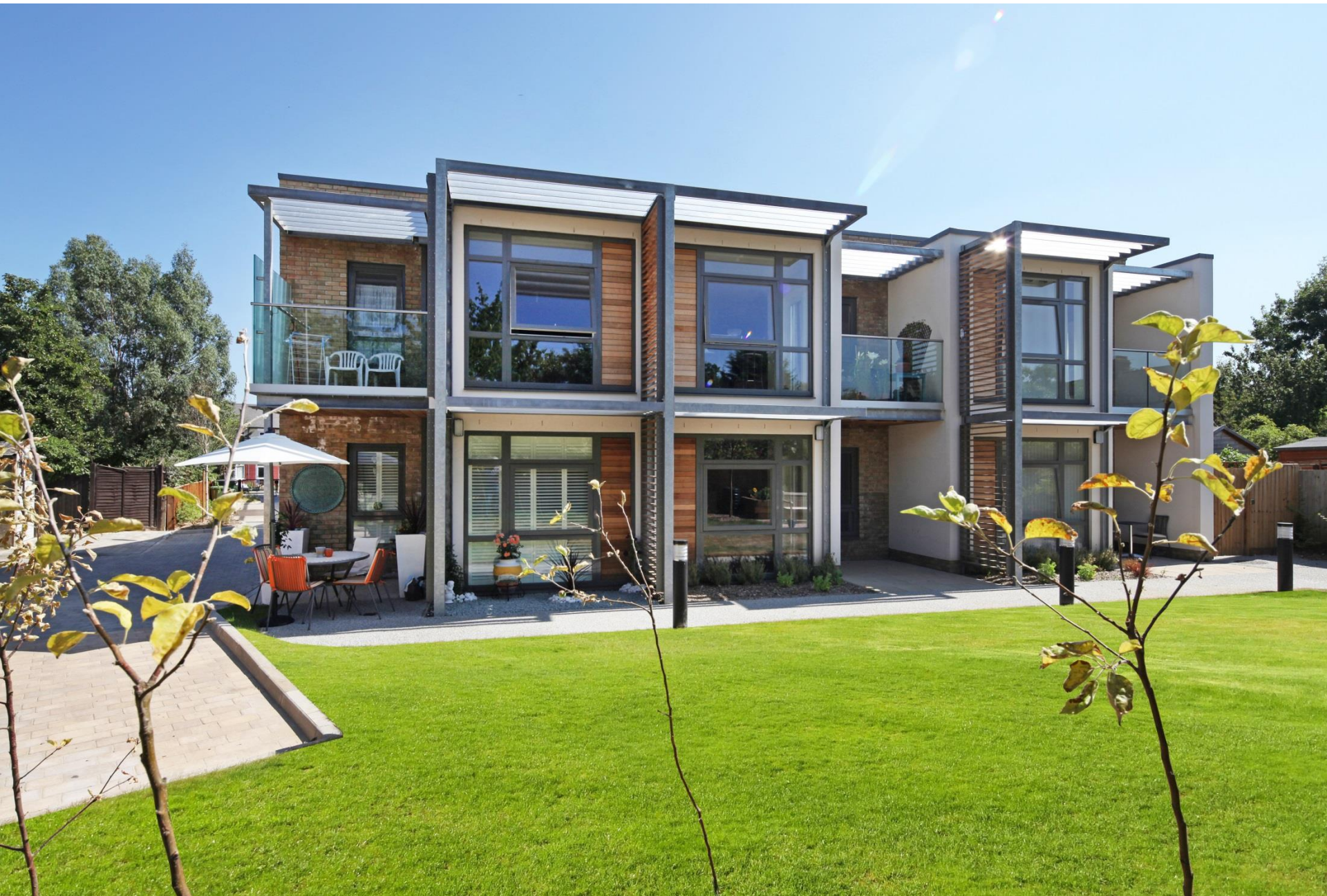
Gresham House, New Malden
