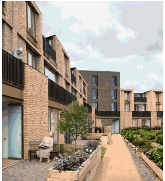
External view showing the wheelchair apartments fronting onto the shared courtyard garden.
