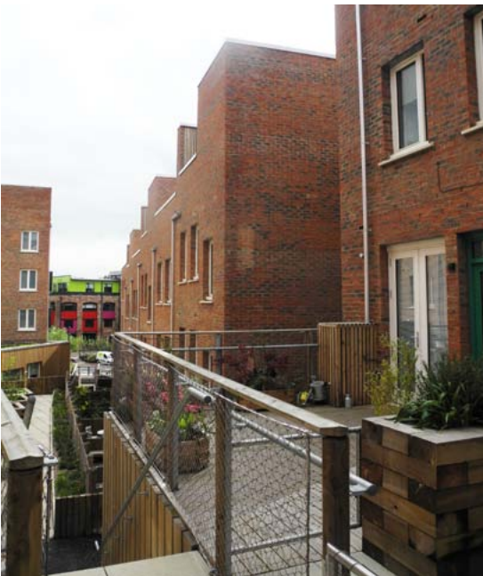
Front yard gardens and shared growing spaces give residents an excuse to be outside and be seen. Malings development in Ouseburn - designed by Ash Sakula and developed by Carillion Igloo.
