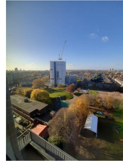
Walter Tull House: Bespoke Housing programme Target: 6 Engage: up to 6 for deployment
