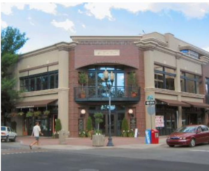
Extract from design code: how a street corner building should orient the primary entrance to the corner.
