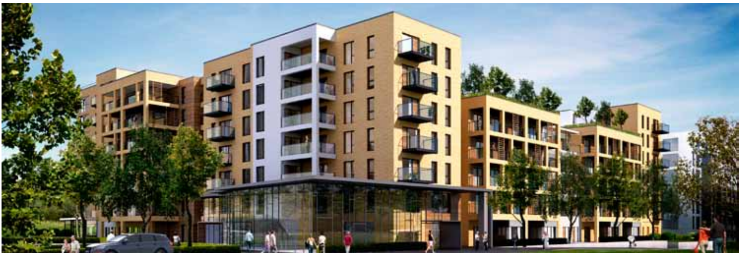
The attractive contemporary design provides generous sheltered balconies to all apartments, many of which are dual aspect. Extensive communal facilities are provided at the ground floor which are designed to enable access by the wider community to create a 'community hub'.
