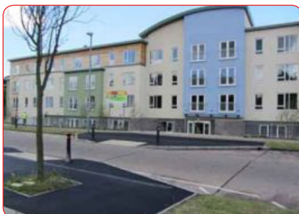
Westhall Court, Birmingham
